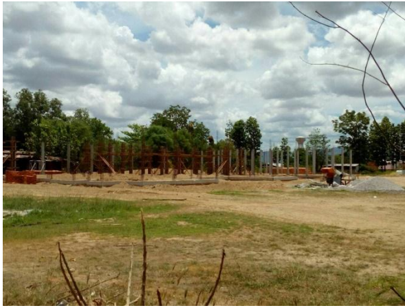
Plate 1 Construction site of Shwekokko (25.4.18)
